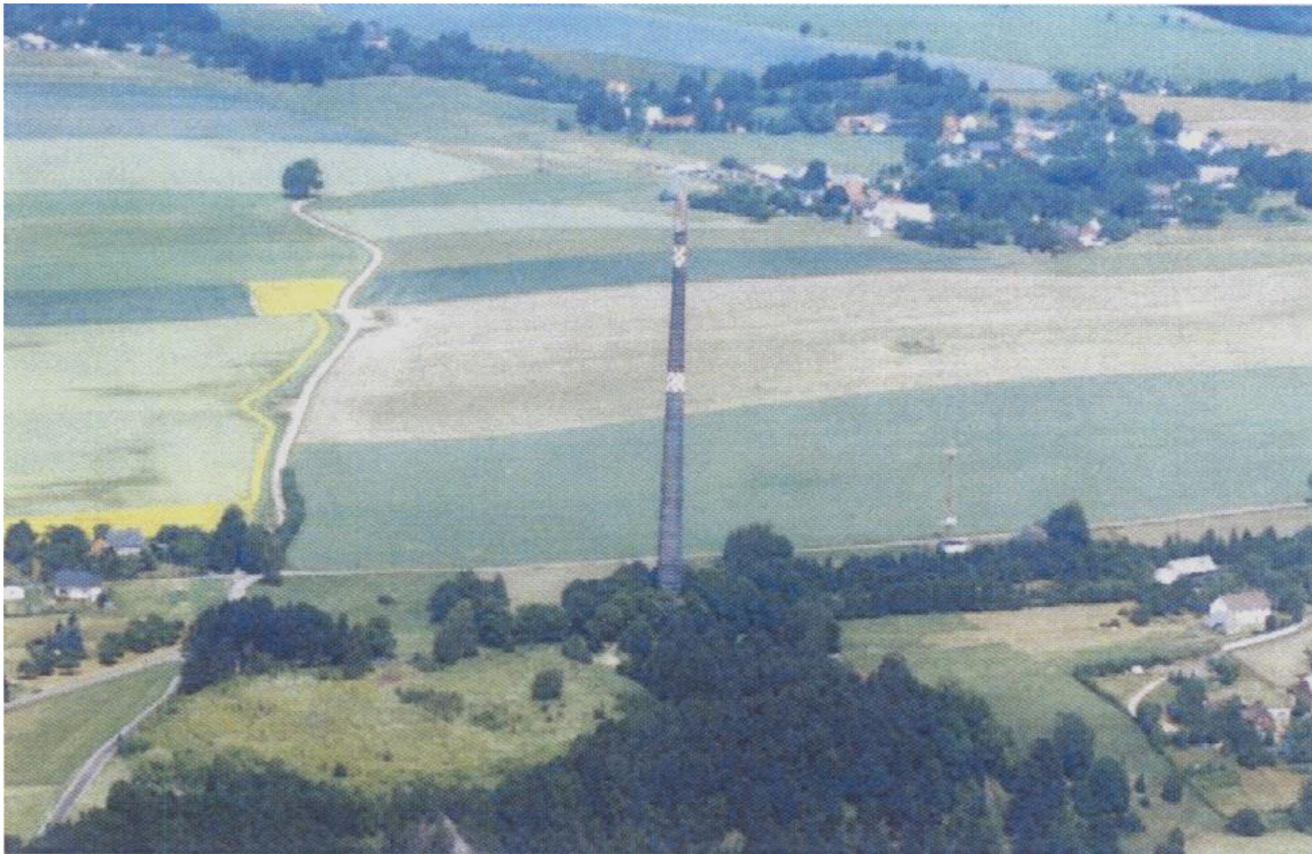
Hohe Esse Halsbrücke (Freiberg, Saxony, East Germany)
